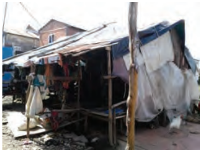
A shanty house built on the given plot of land at a resettlement site in Andoung Chas, Andoung village, Sangkat Kouk Roka, Prek Pnov District, Phnom Penh. Photo: Cufa
