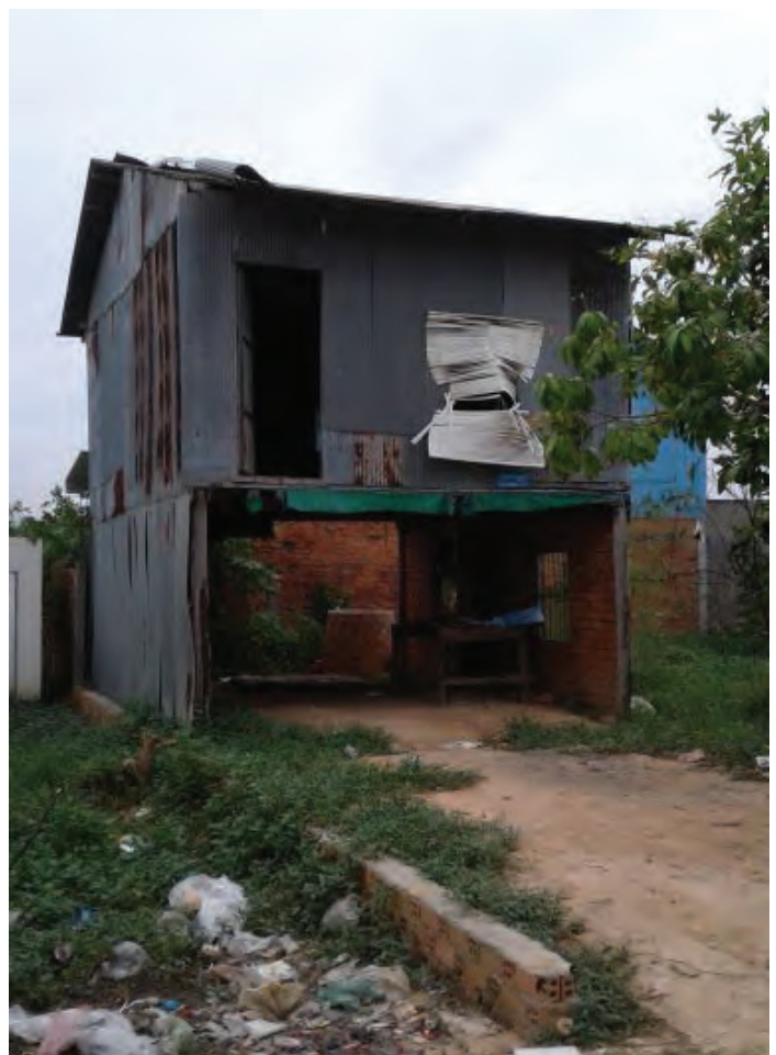
Caption: This photo shows an abandoned house at a resettlement site in Trapaing Anchach Thmey, Phnom Penh. Photo: Cufa
